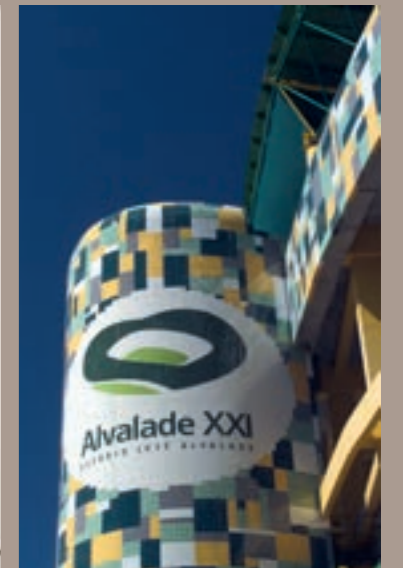
Estádio Alvalade XXI (Sporting Clube de Portugal) — Arq. Tomás Taveira Alvalade XXI Stadium (Sporting Club of Lisbon) — Tomás Taveira, architect
